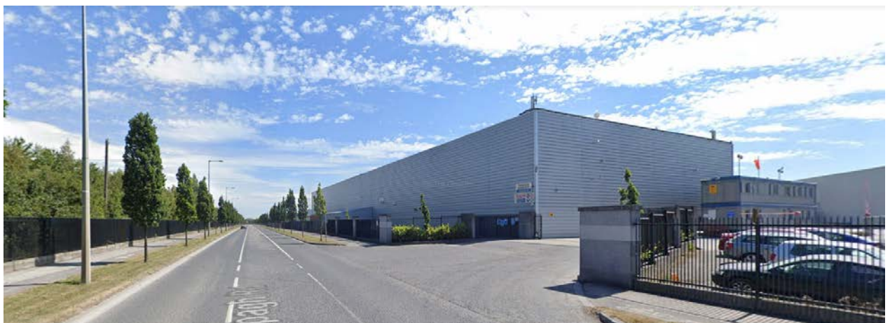
Figure 3.4 – Site 4: Cappagh Road access to Panda facility (Source: Google Maps)
