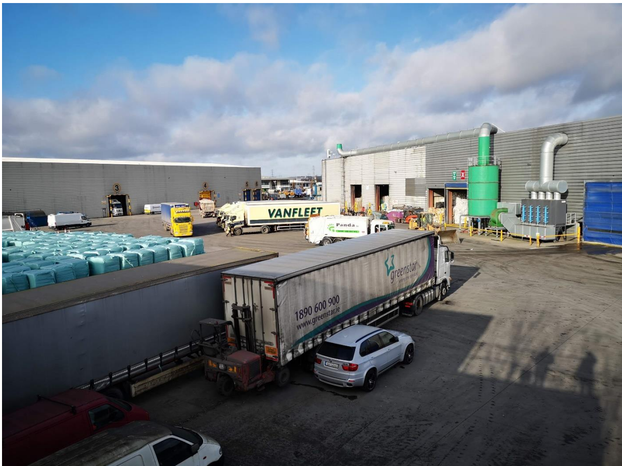
Photograph 12.1 Buildings A1, A2 (Right) and B1 (Left) and yard (Foreground)..
