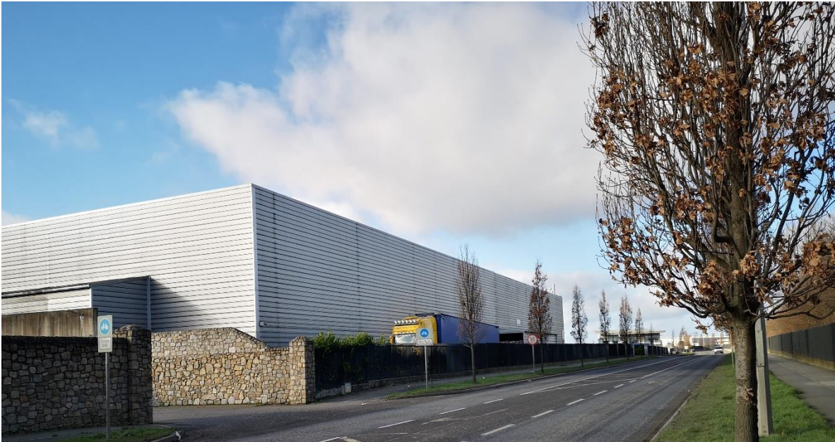
Photograph 12.7 Approach from South
