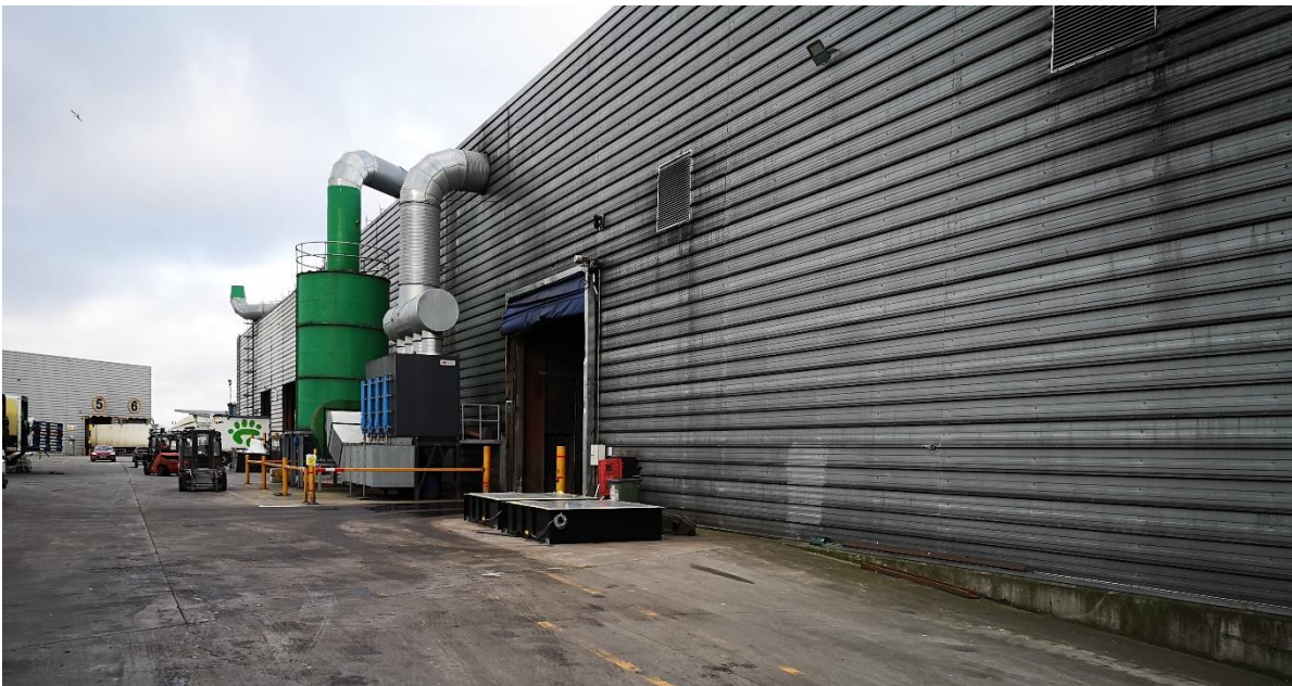
Photograph 12.3 Western Elevation of Building A1 and A2
